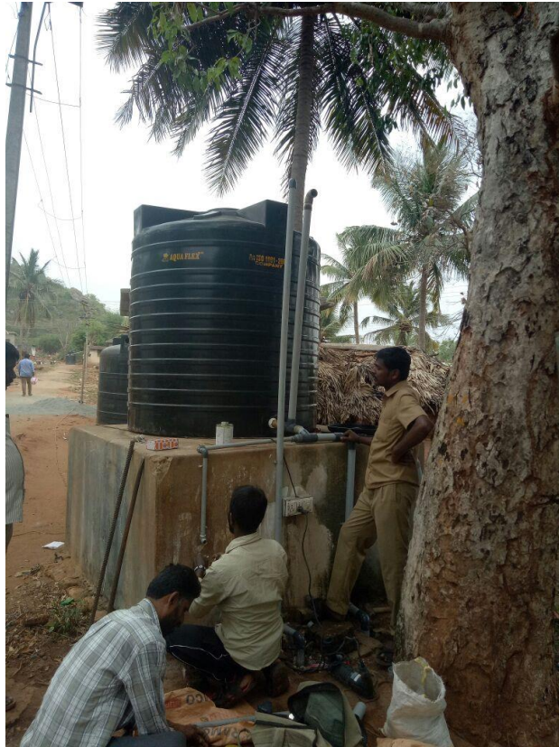
PLUMBING WORK IN PROGRESS
