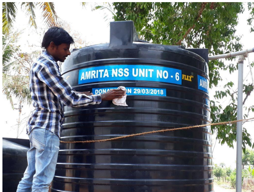
TANK ERECTION COMPLETED AND FULLY OPERATIONAL (29.03.2018)
