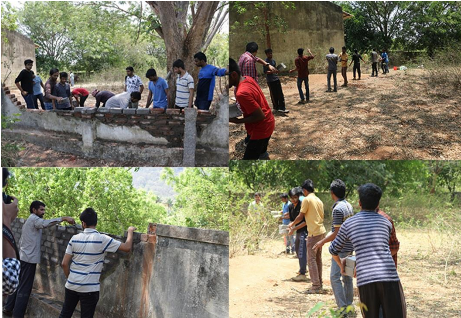
Repairing of compound wall for a tribal school at Chinnampathy by NSS volunteers
